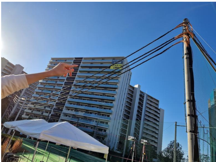
363m aerial cable
