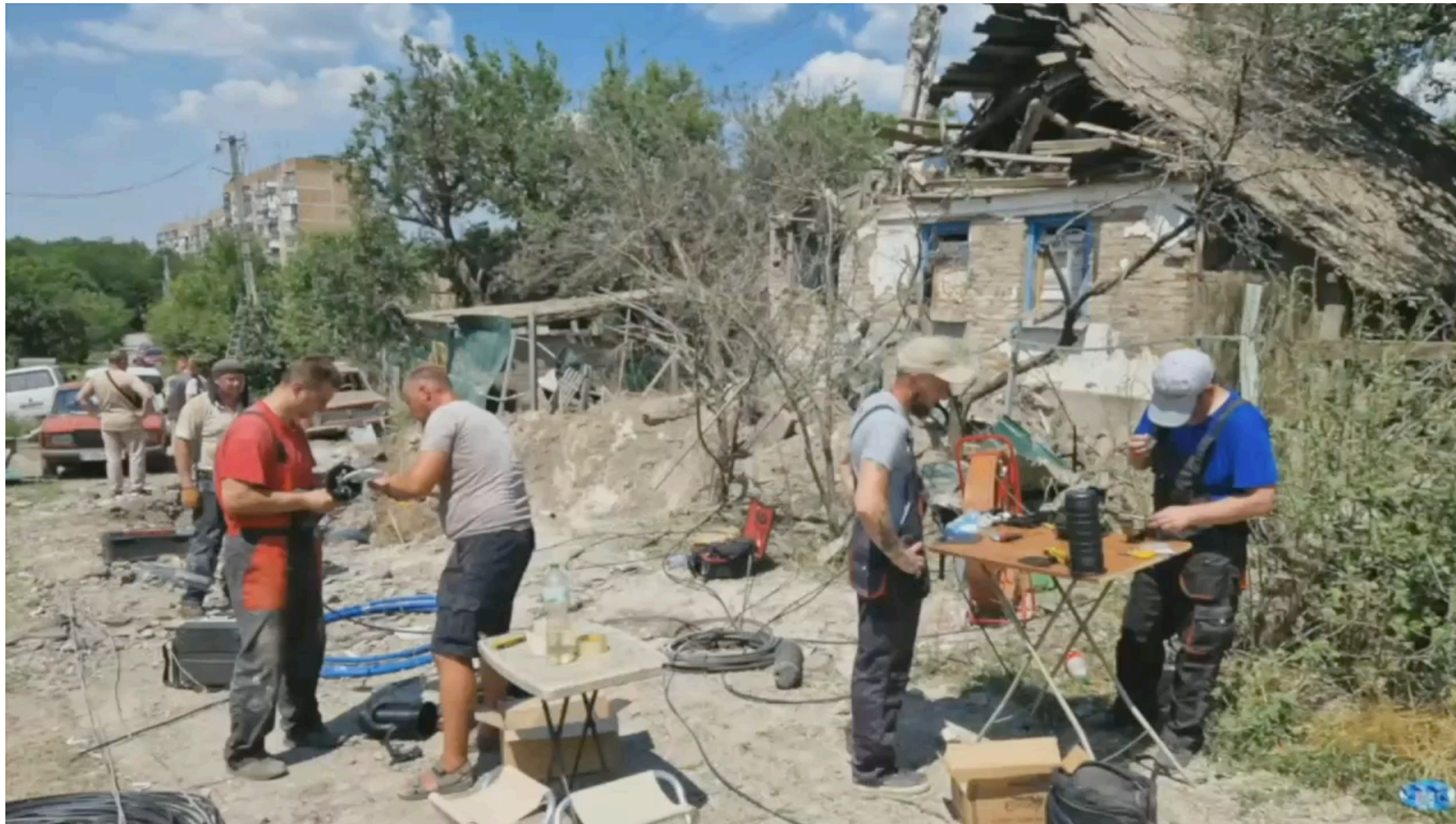
Repairing damage from Russian attacks in Ukraine Source: https://ripe90.ripe.net/archives/video/1582/
