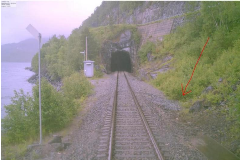
Rockfall 10 m before railway
